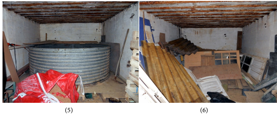
Figure 13. M134 (21)-(1) entrance with concrete access ramp and protection walls, (2) M134 plan: 4 ammunition room (Rudi 1988), (3) corridor with ammunition room entrances and metallic ceiling, (4) room door, (5) ammunition room, (6) ammunition room.
